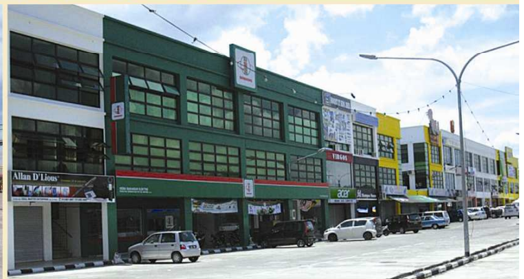
Newly Completed 3-Storey Shophouses (Phase 2)
