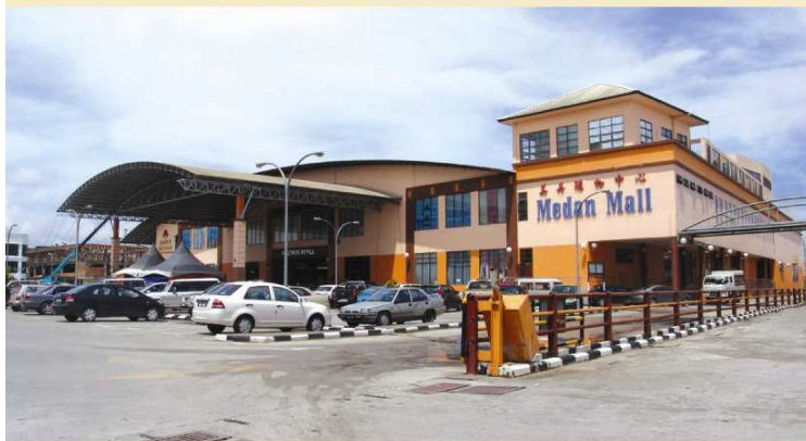
Existing Medan Mall Shopping Centre
